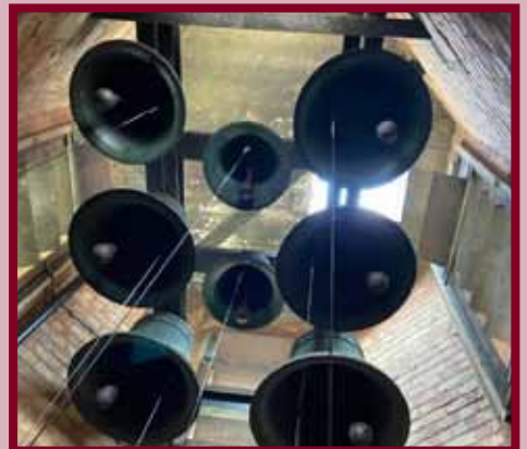
The bells of St Polycarp's Church, Finaghy, were rung for the first time in three years on August 9. They had been out of action as some of the wires attaching the pull hammers to the bell mechanisms were ready to snap. Thanks to generous bequests given in remembrance of two long-time parishioners, Sallie Kenwell and Dawn McConnell, the necessary works were successfully undertaken.
