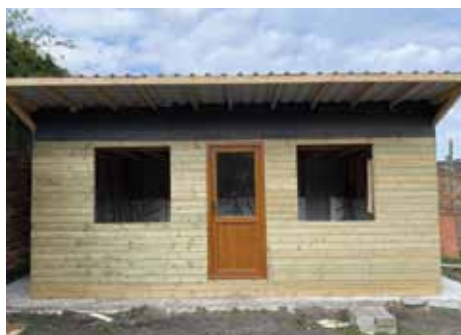
The community cabin taking shape during May.
